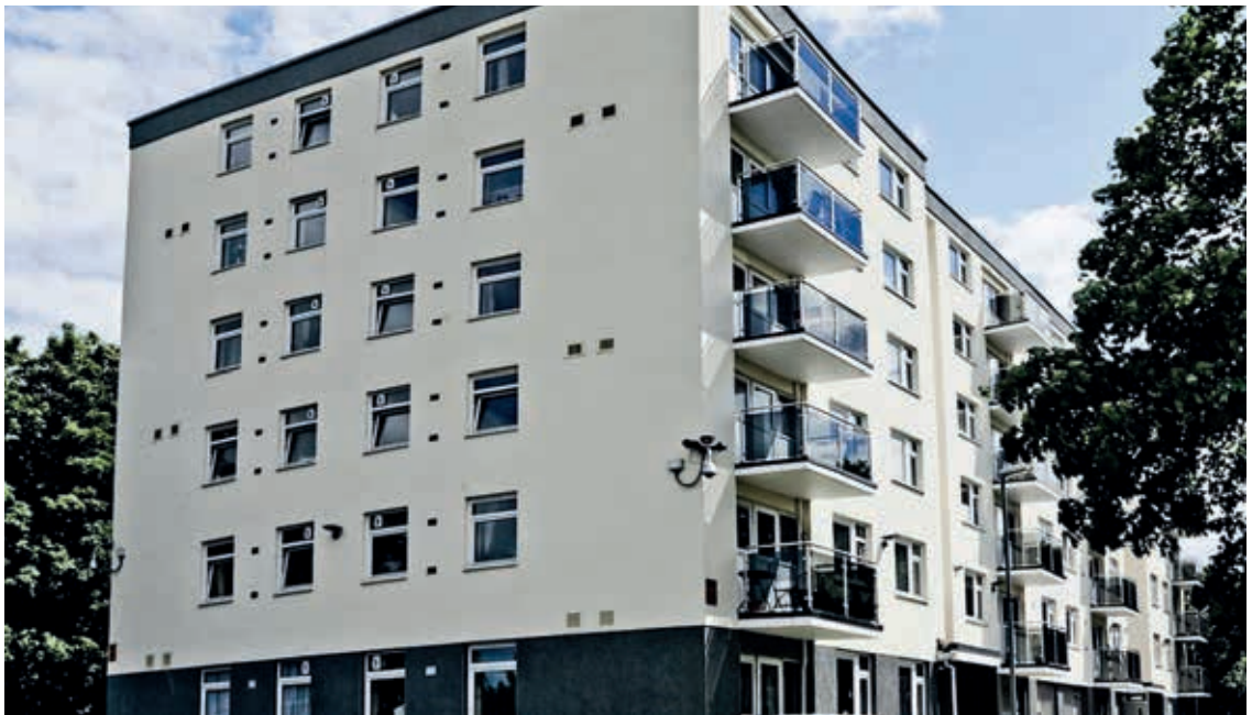
FIGURE 15 Typical residential sector refurbishment project © CMS
